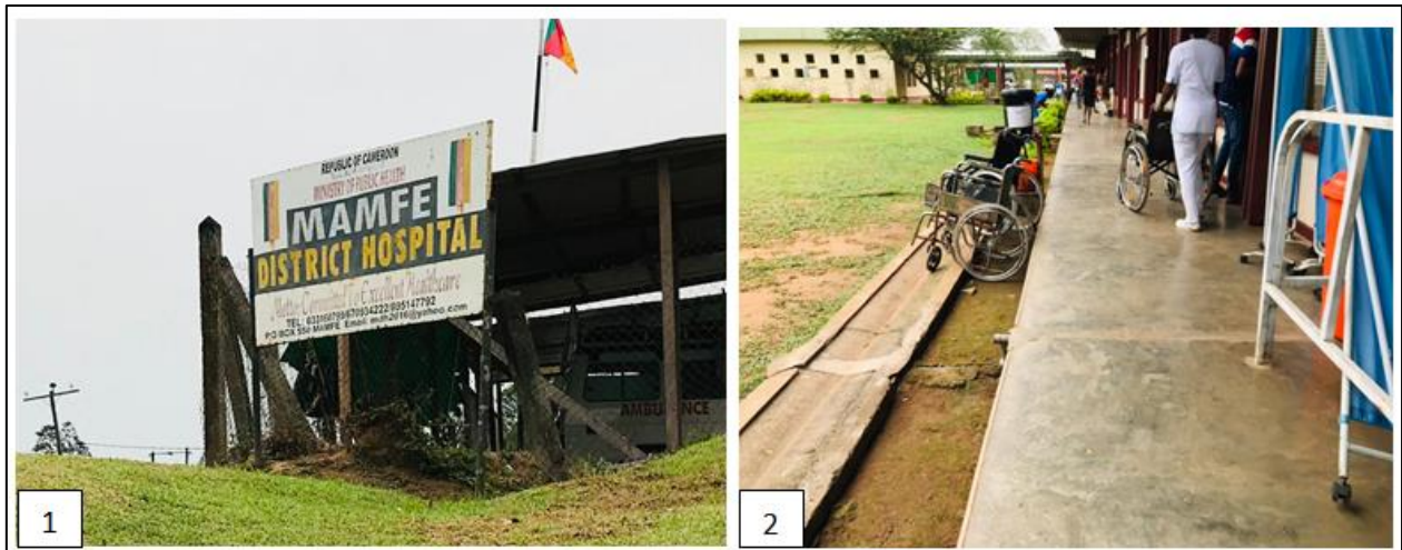
Plate 1: The Mamfe District Hospital resulting from the high way construction Enow, 15 th November 2021
