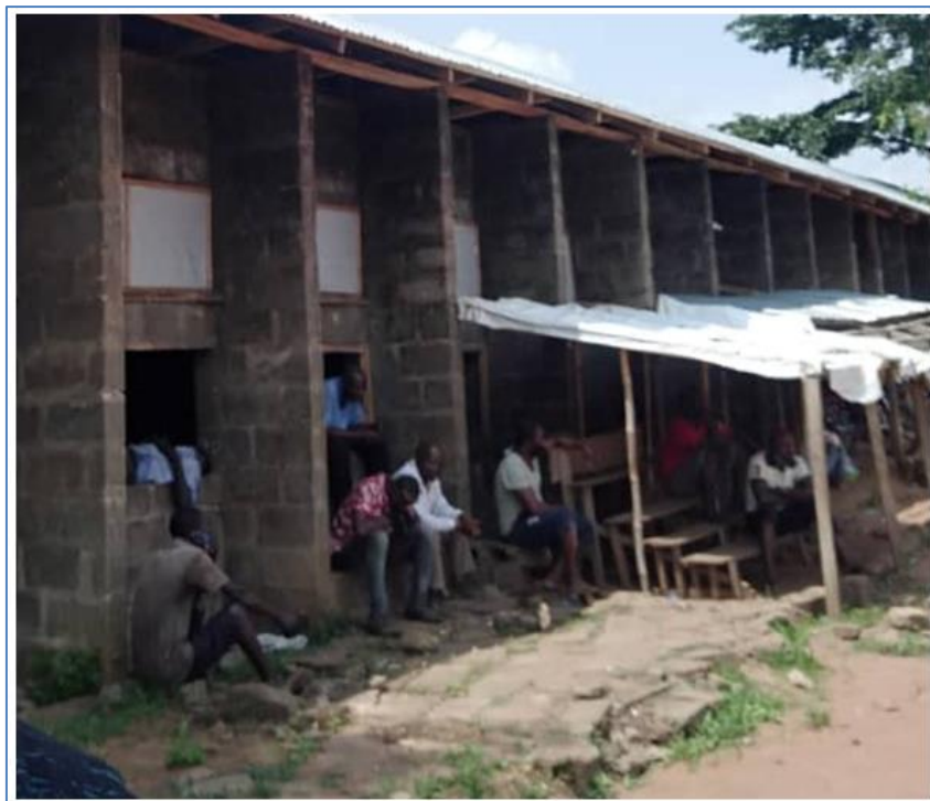
Figure 3: Refugees relaxing in an uncompleted building in Okende settlement
