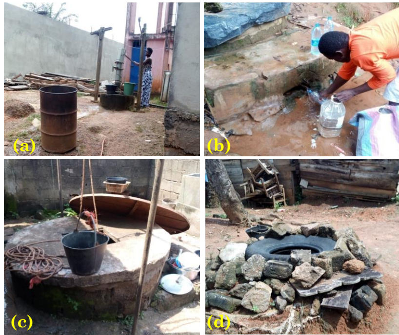
Figure 5: Alternative water supply sources in Yaounde III Subdivision. (a) Drilling; (b) Spring; (c) Protected well; (d) Unprotected well Source: NIMPA Tatiana, 2018
