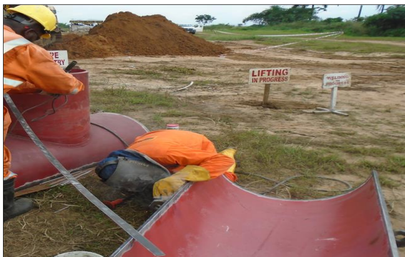
Figure 7: Pipe Sleeve Preparation
