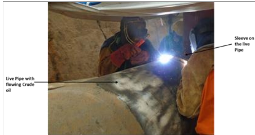
Figure 8: Buttering Layer Welding
