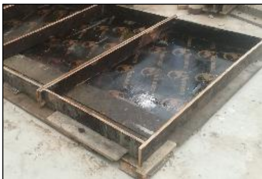
Figure 5: Formwork used for slabs
