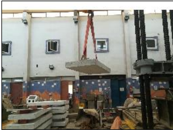
Figure 11: Transported of slab
