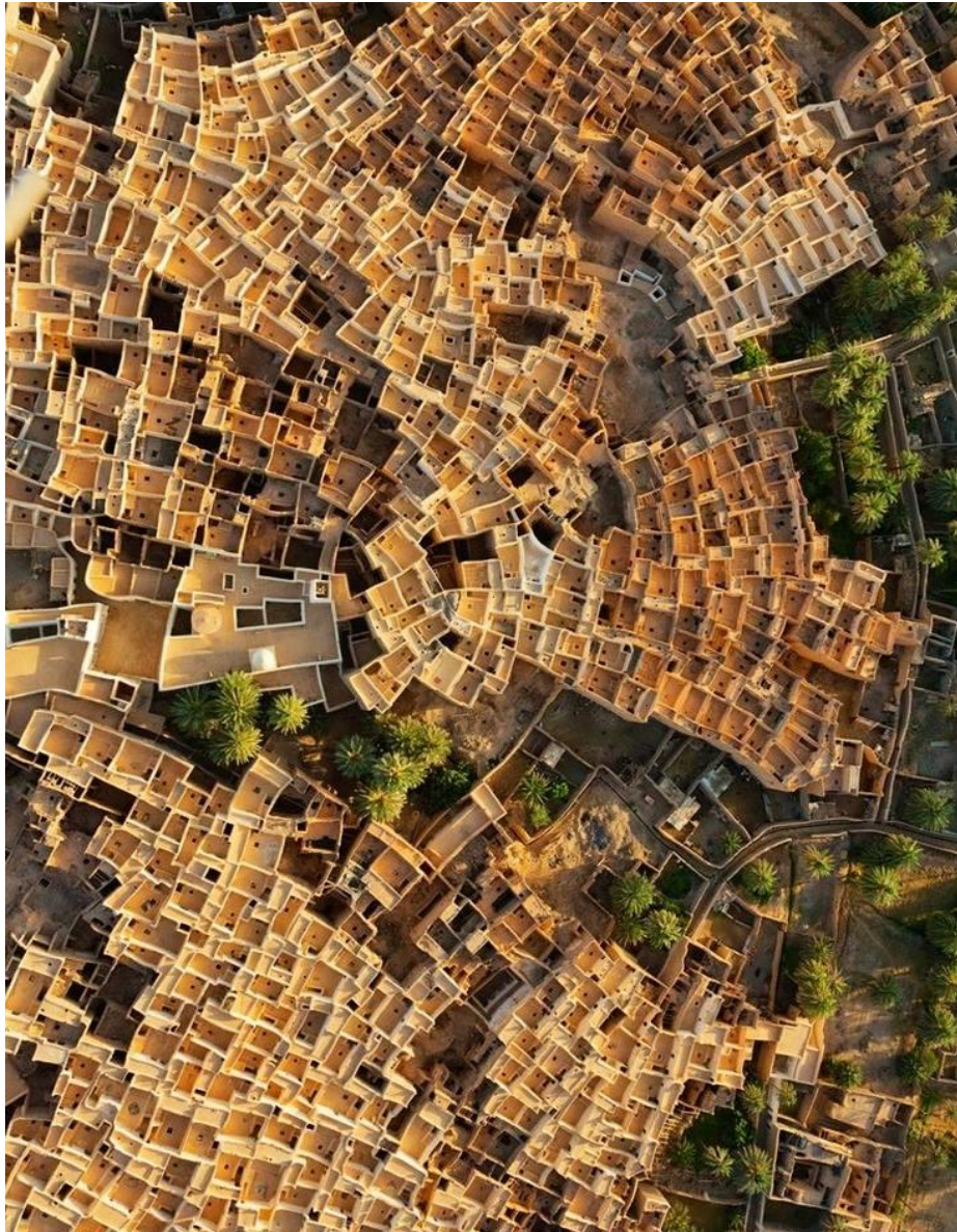
Figure 11: Built in the desert areas where very high temperature in the western of Libya. Design is based on the agglutination building blocks to work with some of the city and one as a bloc with the environment, using small windows for ventilation top of the wall, built of stone and mud. Top view of Ghadames. Eric Lafforgue photography
