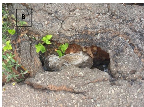
Figure 2: (a) Sinkhole at Awka site 1 (b) Soil pipe at Awka site 2
