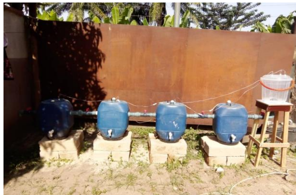
Figure 4: Experimental set-up of the treatment tank
