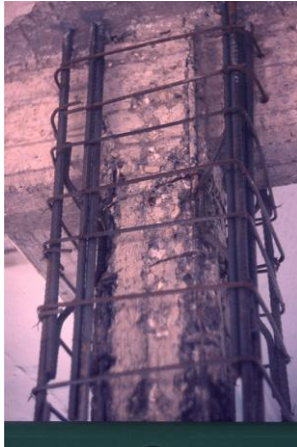
Fig-3: Only two bars bundled together
