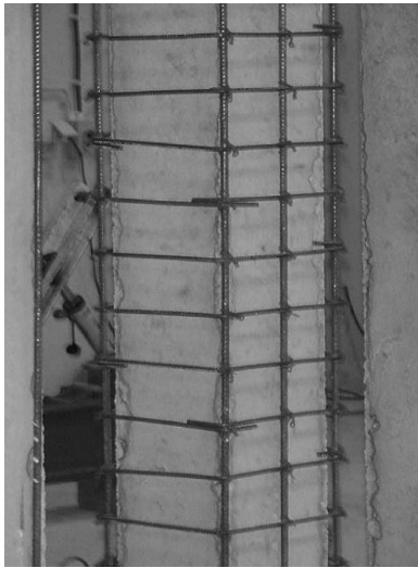
Fig-1: Simple concrete jacketing
