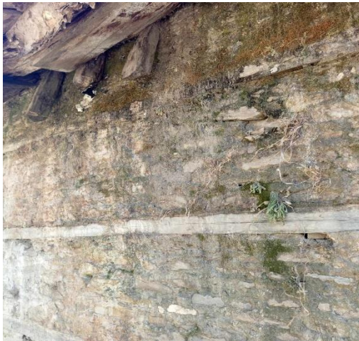
Picture 3: Mud plaster fall down & weathering effect is seen at wall surface
