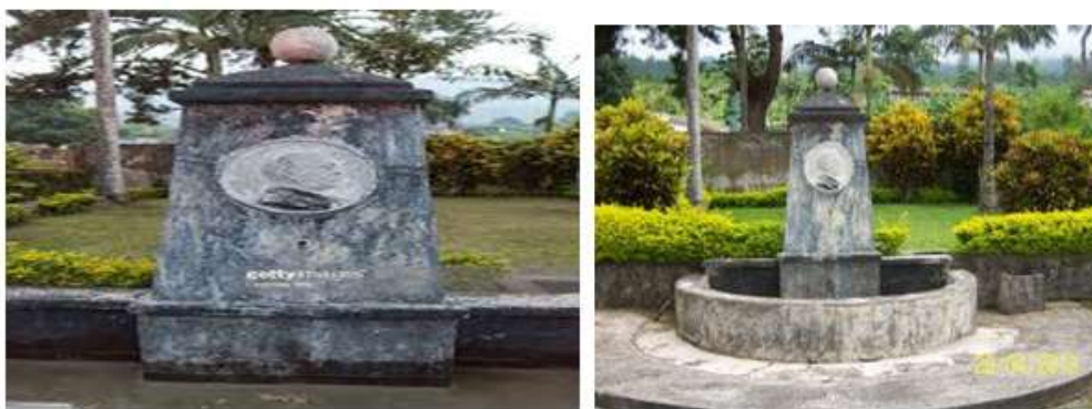
Fig-6a: The BFM before renovation (pre 2009)
