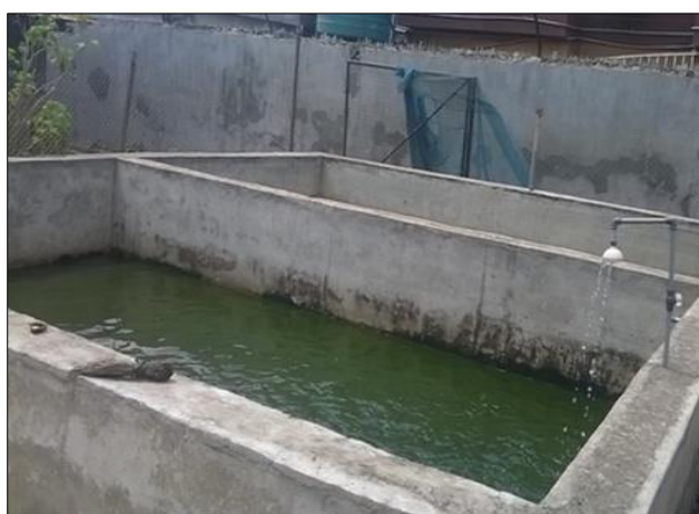
Figure 2: Concrete Fish Pond
