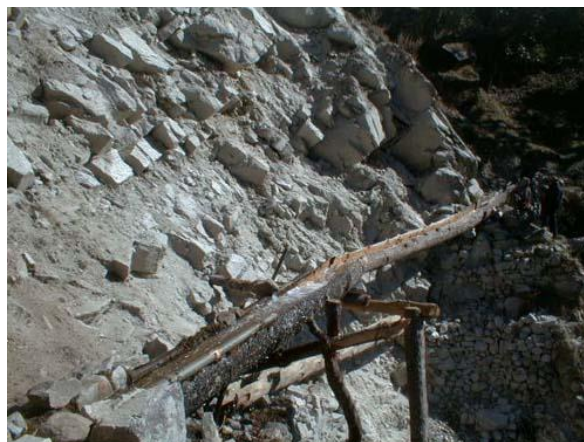
Figure 8: 'Traveling' inside by dangerous areas (Chilkhaya, slide crossing with wooden aqueduct, Nepal, 1999-2001)
